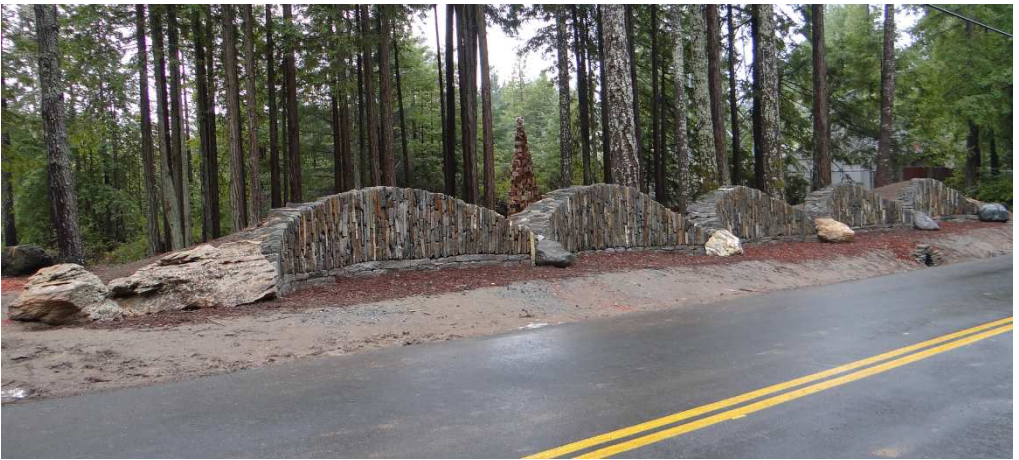
Fig 12. The completed wing wall
