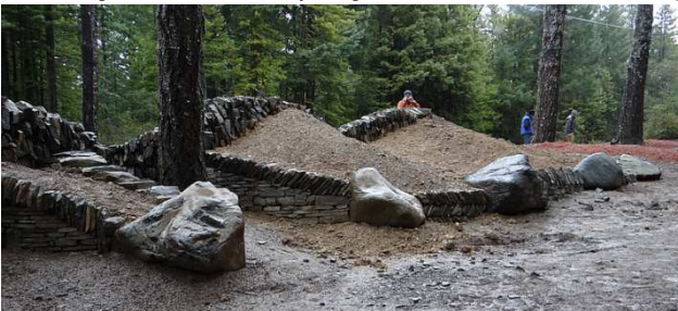
Fig.14. Back of the Wing wall (1)
