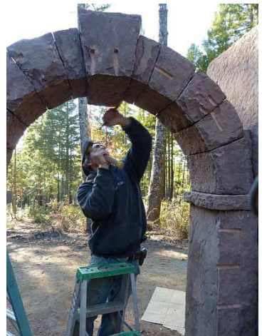
Figs.16. (above) and 17 (below) Setting and working on the keystone Photos © SeanSmyth
