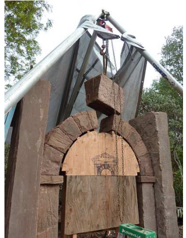
Figs.16. (above) and 17 (below) Setting and working on the keystone Photos © SeanSmyth
