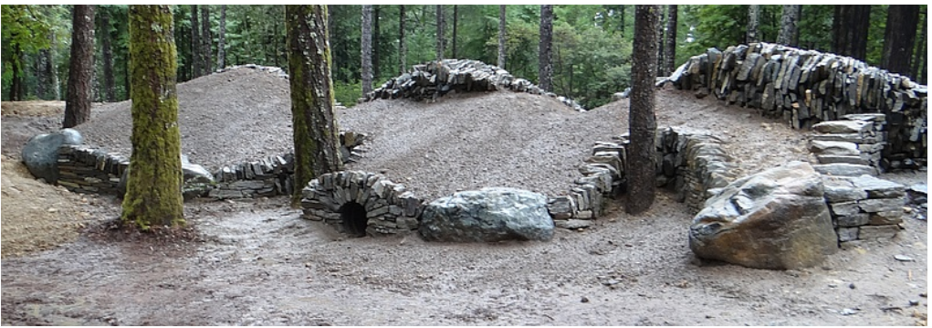
Fig.15. Back of the Wing wall (2)
