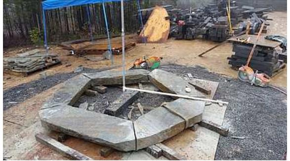
**Fig.7. (Left) The roof dry run in 2 halves. © Sean Smyth**
